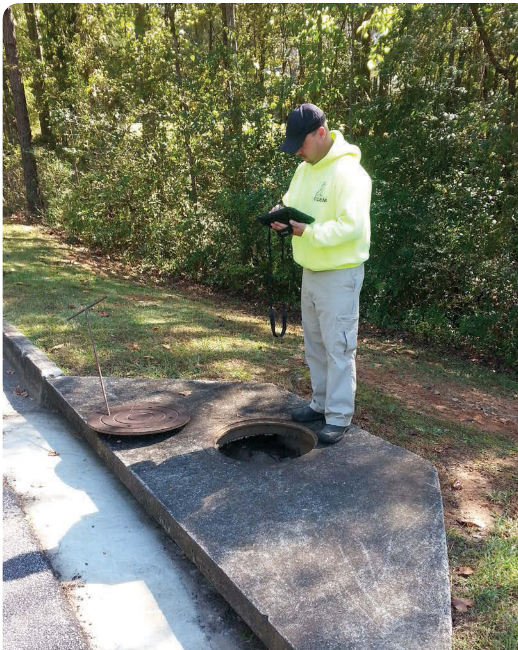
↑ Coweta County field inspector Scotty Truitt inspects a catch basin in a subdivision. Collector for ArcGIS lets him document his findings.
