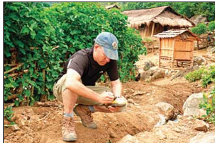
GPS data collection along the pipeline in Ban Phakeo Village.
