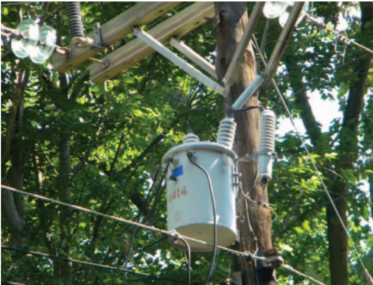
← Field Picture of Single-Phase Transformer (with lightning arrester)
