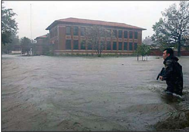
LAFB Flooded from Hurricane Isabel, September 18, 2003
