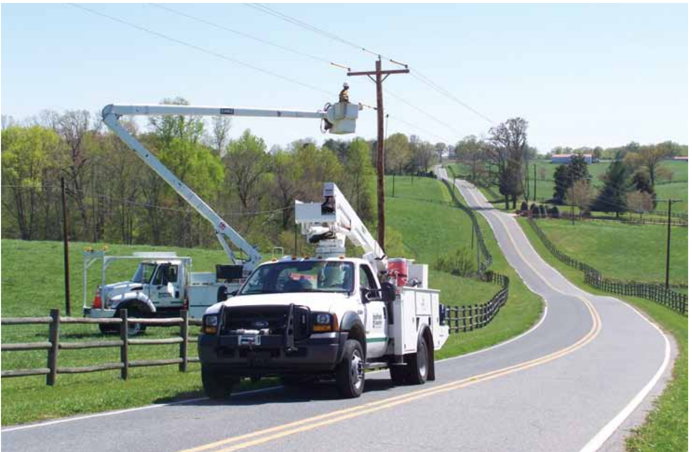
↑ Union Power crews maintain distribution lines.
