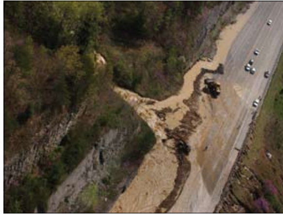
A mine blowout in Knott County, Kentucky, resulted in the closure of KY 80, a four-lane highway connecting Hazard and Prestonburg. The blowout was quickly located with the help of the KMMIS mine map database.
