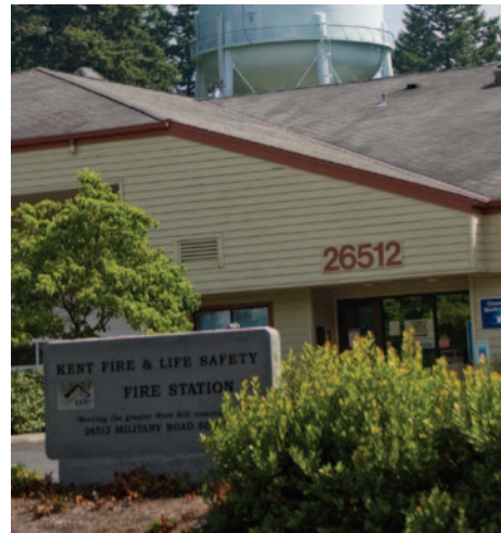
Kent Fire Station 73, located in the southwest corner of the district, protects residential and commercial occupancies along a major interstate highway.
