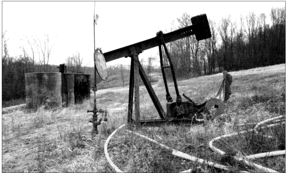
↑ A Pump Jack, Production Equipment, and Tanks That Were Found during a Field Inspection
