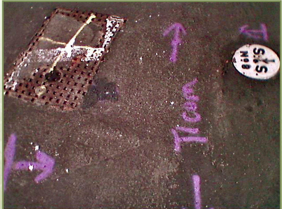
Figure 7.8 Asset repair ground markings.
