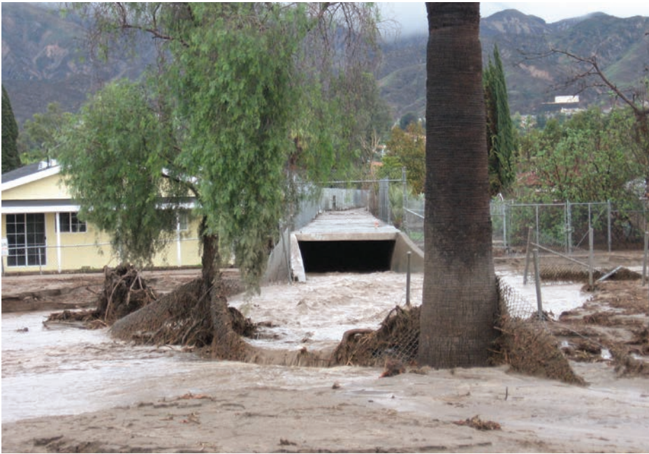
↑ An outlet of a flood control facility has overflowed and pours mud and water onto city streets.
