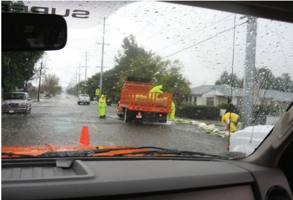
↑ County flood control crews sandbag a location to prevent further flooding of private property.
