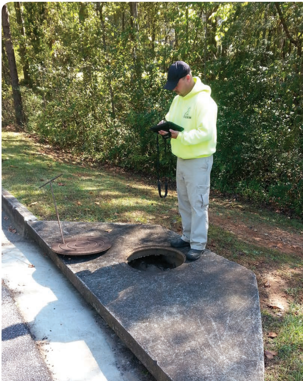
↑ Coweta County field inspector Scotty Truitt inspects a catch basin in a subdivision. Collector for ArcGIS lets him document his findings.
