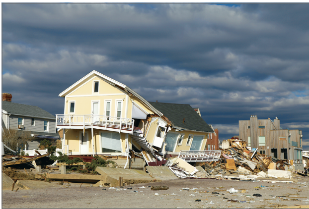
Figure 1.34. Homes destroyed by Hurricane Sandy in Far Rockaway, New York, in 2012. Many people perceive natural hazard risk as minimal, and they continue to build in places prone to hurricane wind and flood damage. Photo by Leonard Zhukovsky. Stock photo ID: 130759928. Shutterstock.
