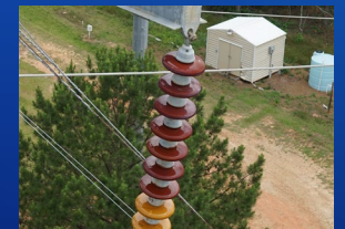
Drone close range inspection
