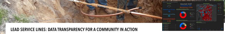
The City of Benton Harbor's water distribution system is more than 100 years old. Water leaving the city's water plant doesn't have lead in it; however, many of the water service lines from the property line to the homes are made of lead or have lead components in them, as do some public-side water service lines.
