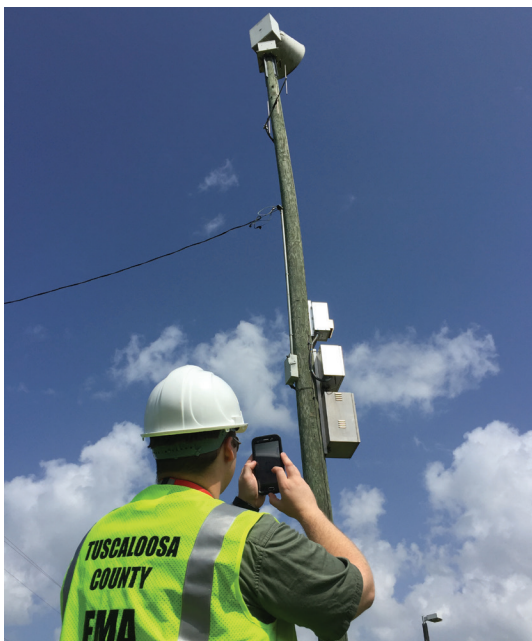
↑ Using Survey123 for ArcGIS, TCEMA specialists can check a siren's location on the agency's existing map at the same time that they conduct a siren inspection.
