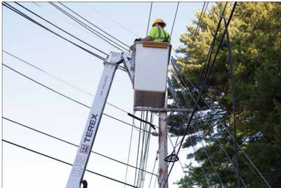
↑ Maine Fiber Company oversees 1,100 miles of fiber network.
