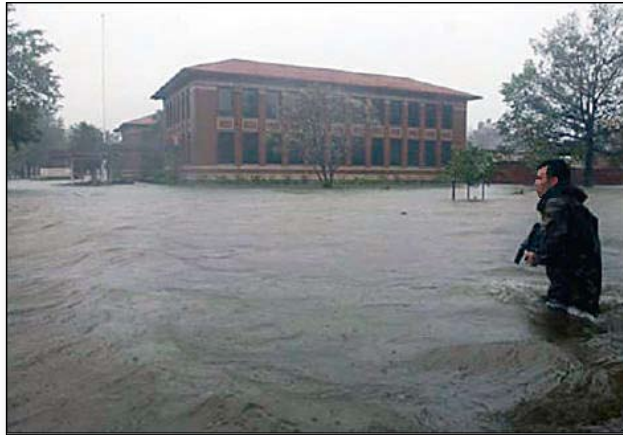
LAFB Flooded from Hurricane Isabel, September 18, 2003
